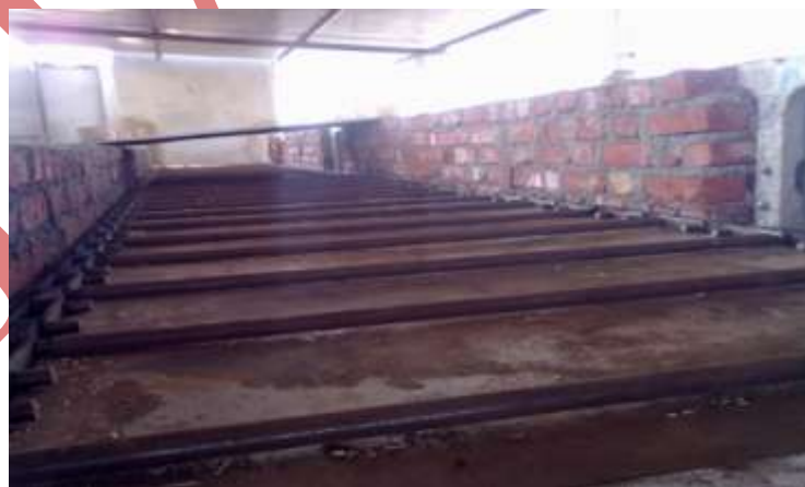
Fig 3. Actual construction of chain conveyor
