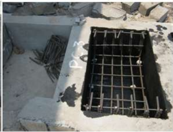
Fig. 11: Plate 4: Reinforcement cage of PB2
