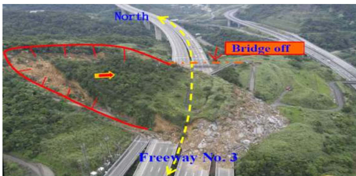
Fig.2 Large-scale landslide of dip slope at 3k + 100 of Freeway No. 3
