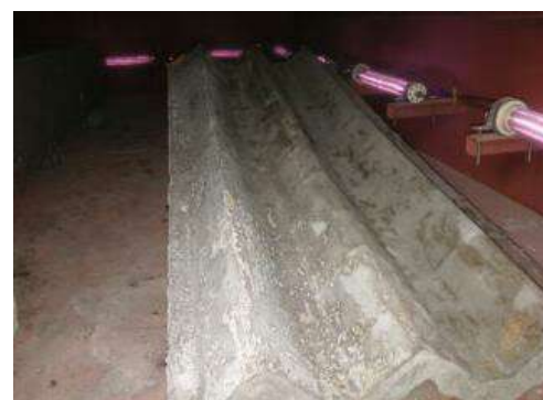
Fig:6 Curing Of Panel In Heat Chamber
