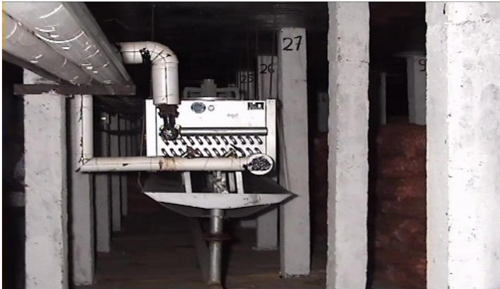
Fig.2 Evaporator located on the Bottom
