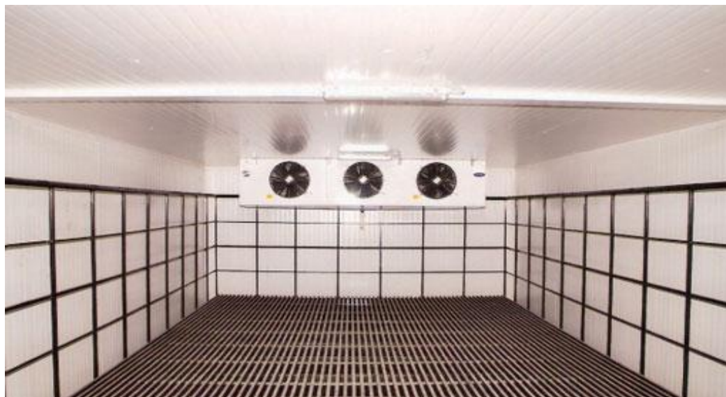
Fig.1 Evaporator located on the Top
