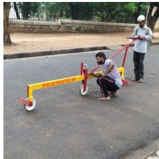
Figure 7 Rolling Straight Edge (RSE) Measurement in Progress
