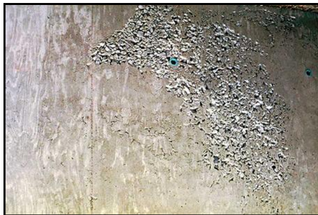
Fig.5 Segregation on removal of formwork
