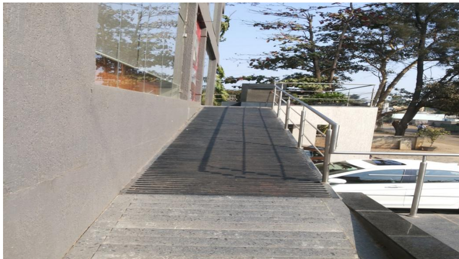
Figure 4 Non slippery ramp
