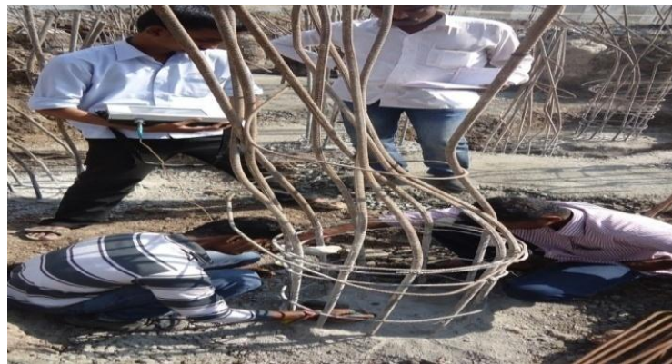
Fig. 7: Pile Integrity Test in progress
