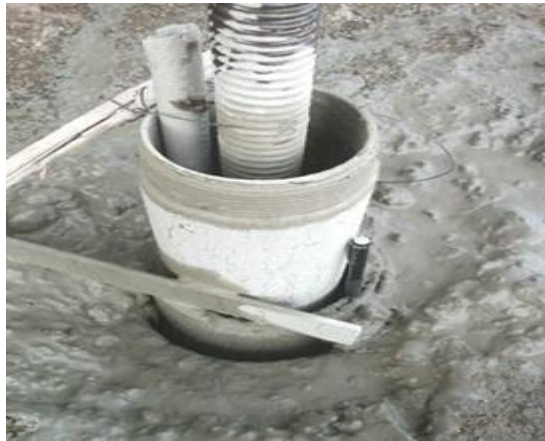
Fig.16 : Installed micro pile.
