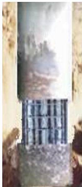
Fig.12. defective pile ready for repairing.
