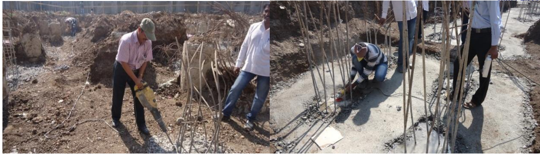
Fig. 5: Breaking of damaged pile portion
