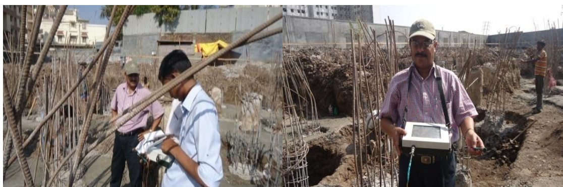
Fig. 3: Pile foundation at Pune Site. Fig. 4: PIT Test Equipment
