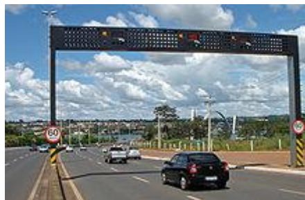
Fig. Automatic speed enforcement gantry or "Lombada Eletrônica" with ground sensors at Brasilia, D.F.
