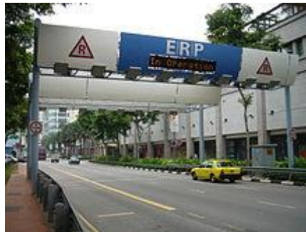
Fig.: Congestion pricing gantry at North Bridge Road, Singapore.
