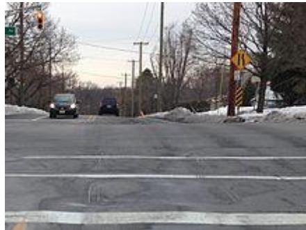
Fig.: Saw cut loop detectors for vehicle detection buried in the pavement at this intersection as seen by the rectangular shapes of loop detector sealant at the bottom part of this picture.
