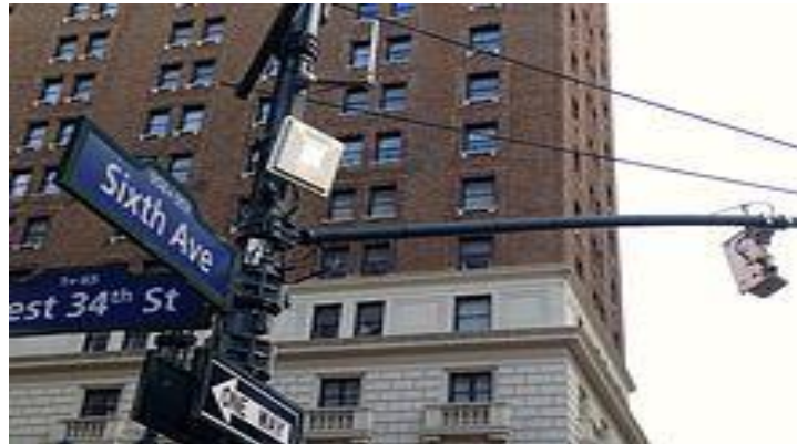
Fig.: RFID E-ZPass reader attached to the pole and its antenna (right) used in traffic monitoring in New York City by using vehicle re-identification method
