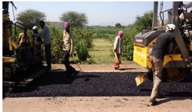
Stabilization with bitumen
