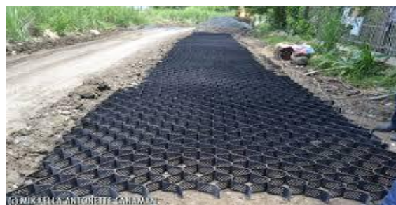
Stabilization with geo-textile
