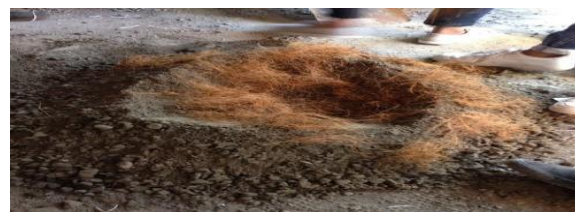
Figure 3 - Mixing of dry concrete with coconut fiber
