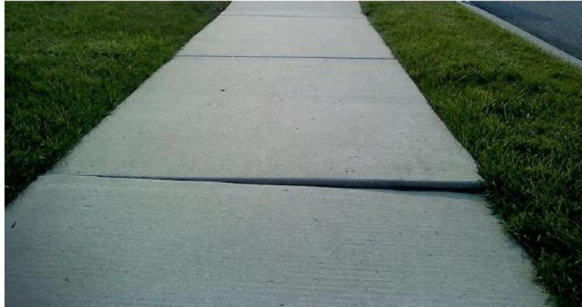
**Figure 5: Uneven Leveling of Concrete Slab**
