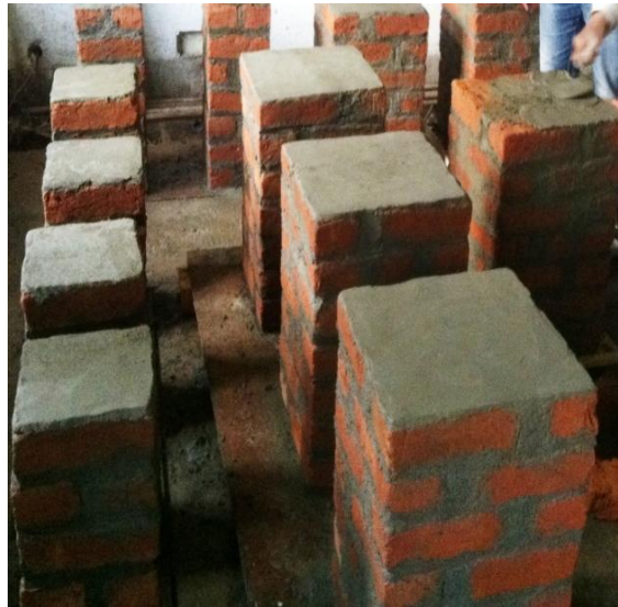
Figure 4.1 (Pictures captured in structural lab during the construction of columns)
