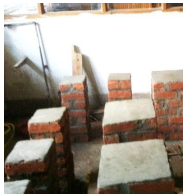
Figure 4.2 construction of pvc confined pcc columns
