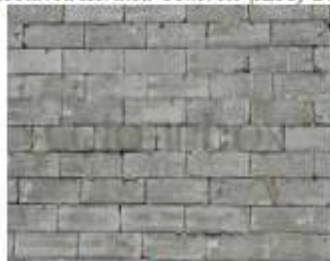
Fly Ash Brick Wall
