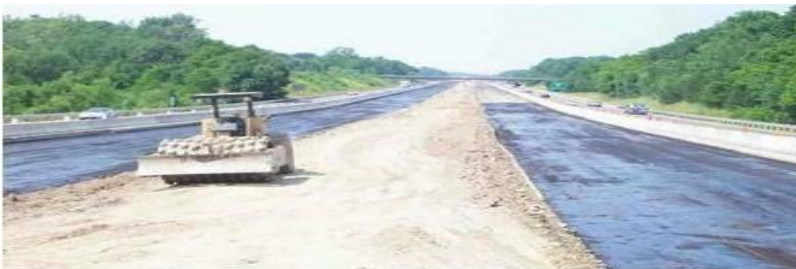
Fig. 7 Prime coat emulsion for curing
