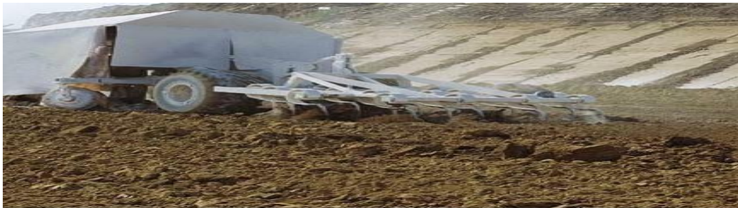
Fig. 2 Scarification before lime application
