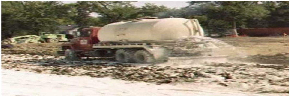
Fig.4 Adding water after dry lime application
