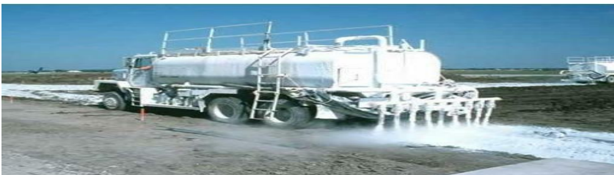
Fig. 3 Spreading of lime over scarified soil
