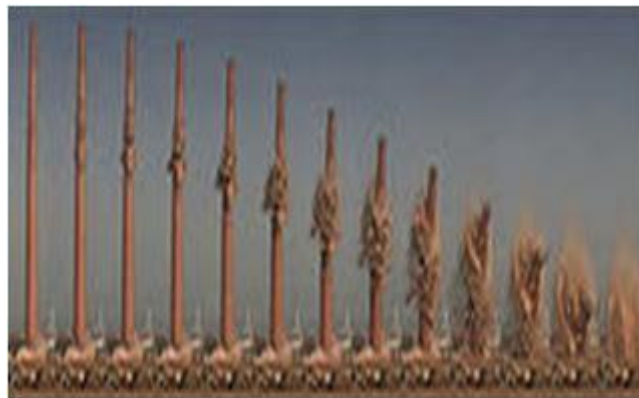
Demolition of a chimney in Germany (falling into footprint)
