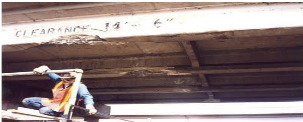
Fig 3.4 Repair and retrofit of concrete structural elements using FRP composites
