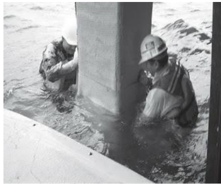
Fig. 4.2 Use of rebar probes in instrumental
