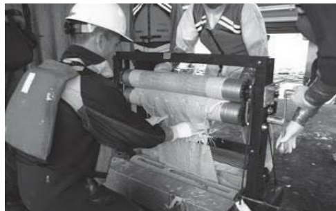
Fig. 4.4 On-site saturation, Friendship Trails Bridge, Tampa
