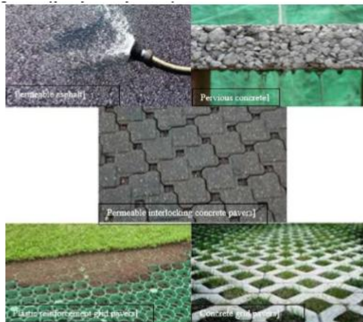
Figure. 2. Figure showing different types of permeable pavement systems
