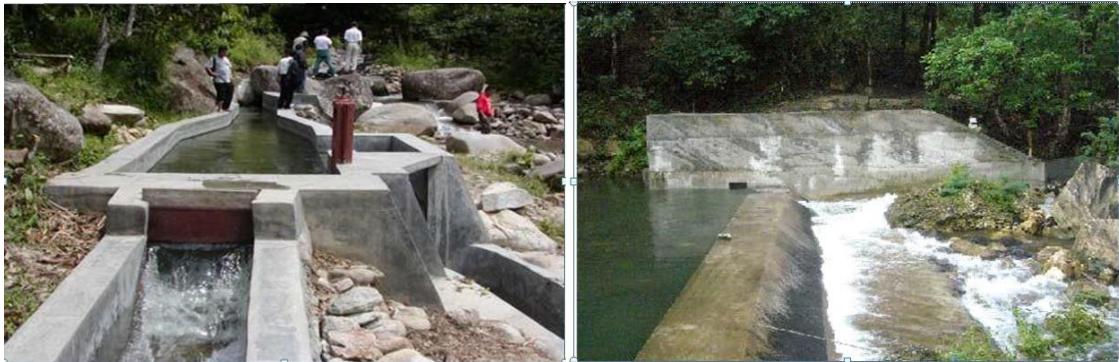
Figure: Settling basin
