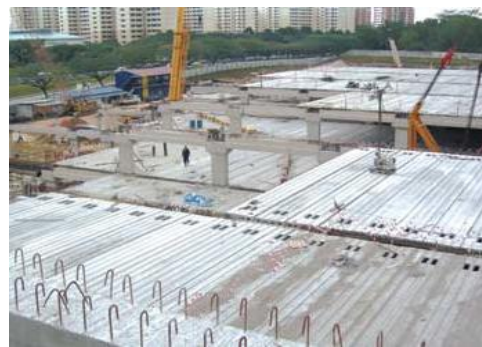
Fig. 3 R.C. Planks laid over partially precast joists
