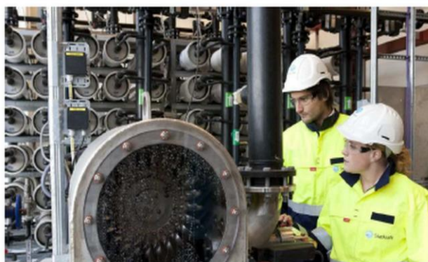
Fig. 5: Pelton Turbine used for Power Generation in Osmotic Power Plant.
