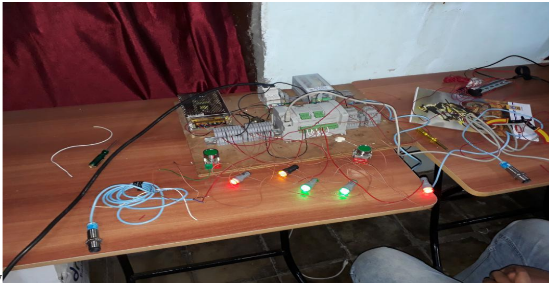
TUNNEL POWER SAVING
