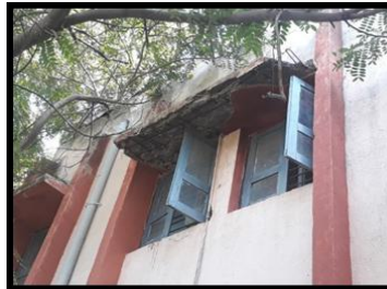
Slab plaster is fallen out and reinforcement is visible
