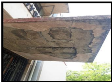
Spalling of Concrete and Excessive Deflection Of chajja
