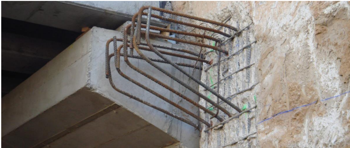
Fig. 4. Visual inspection of structure
