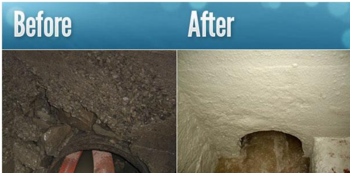
Fig. 7. Rehabilitation of manhole
