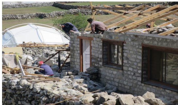
Fig. 2. Reconstruction work after earthquake in Nepal
