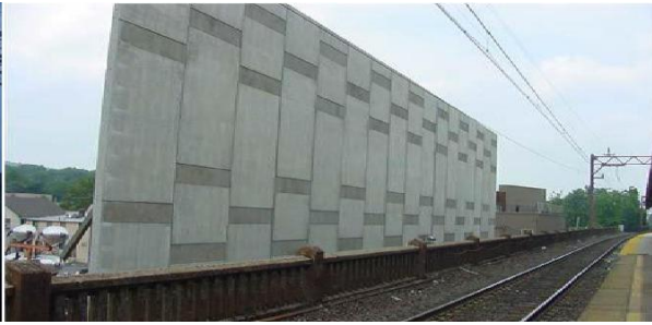
Figure 6 erection of precast wall
