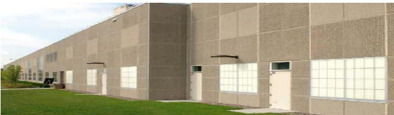
Figure 4 Precast non-composite concrete wall panel.
