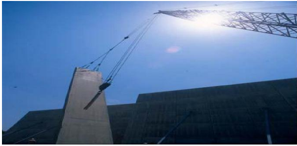
Figure 5 Installation of precast wall
