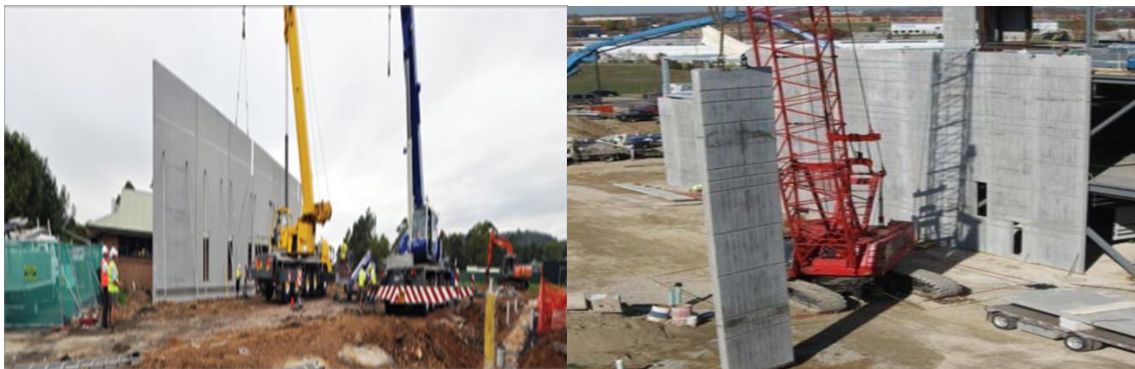
Figure 1: Precast wall panel and Installation of precast concrete wall panel
