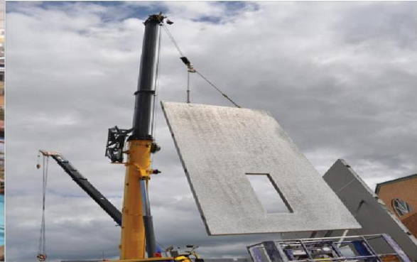
Figure 3 precast wall transport at sit
