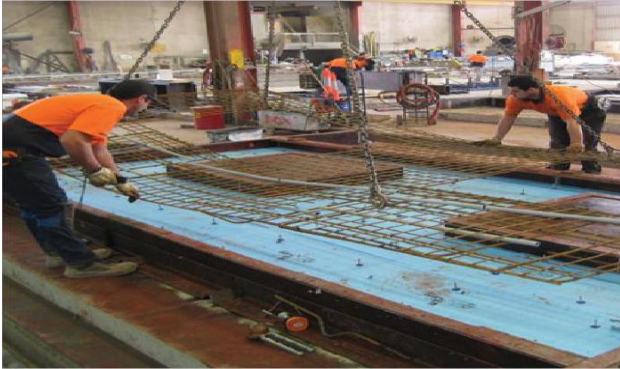
Figure 2 Precast wall casting.
