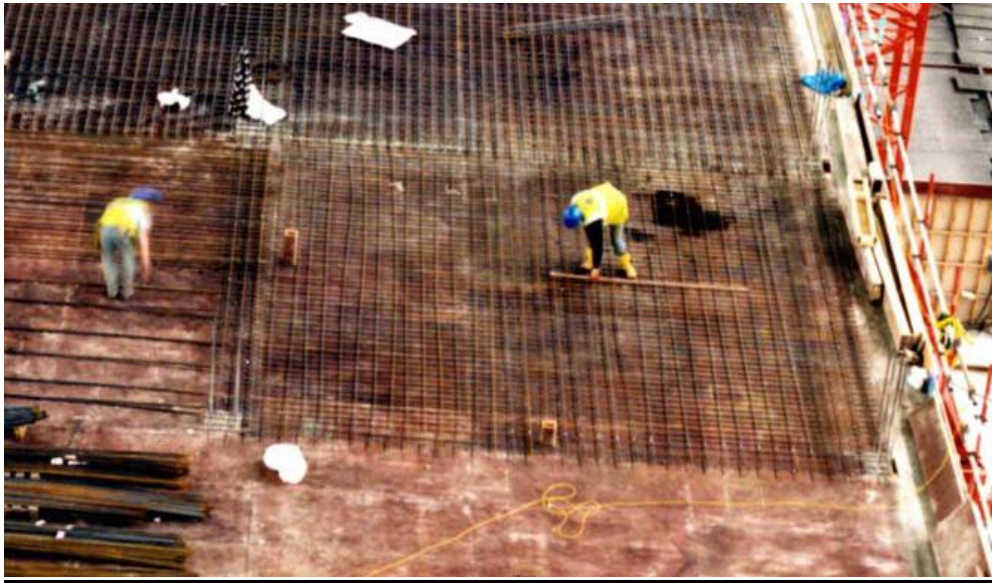
Figure: European Concrete Building Project at Cardington - 4th floor during Construction
