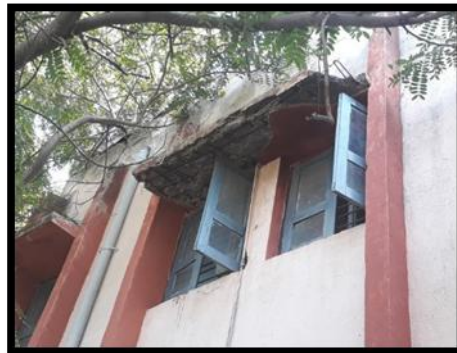
Slab plaster is fallen out and visible
