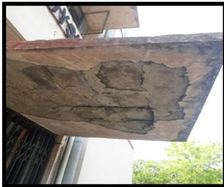
Spalling of Concrete and Excessive Deflection reinforcement is Of chajja
