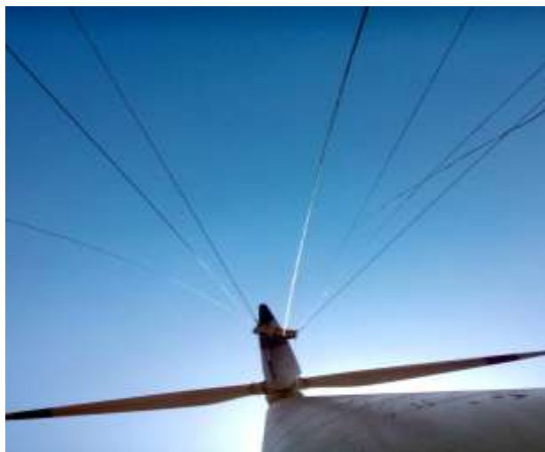
Fig 2: Skylift clamp on hub when hub lock is done
