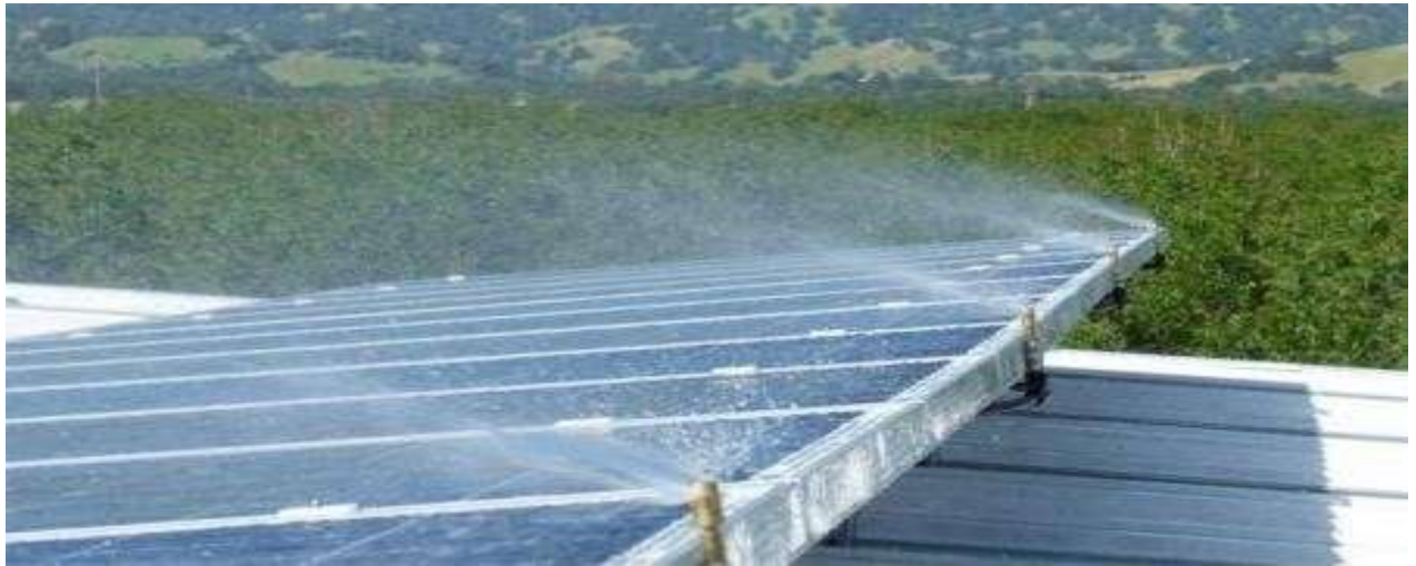
Figure 2-1: Heliotex cleaning technology using water and soap to clean the surface of PV panels.
