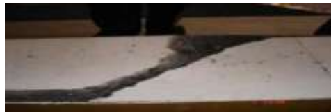
Fig: 1 Failure Patten in pure torsion
